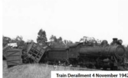
Train Derailment 4 November 1942
